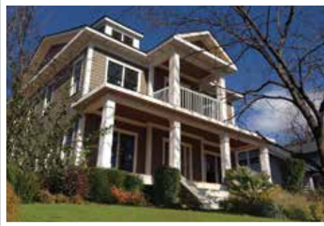
970 DREWRY STREET, VIRGINIA HIGHLAND
